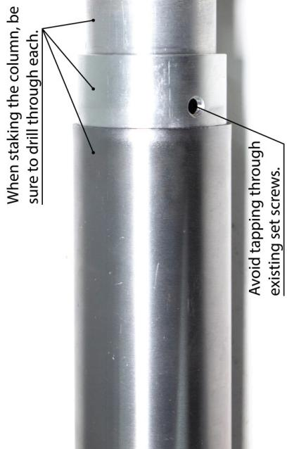
The tapping bolt can go through the column bracket as well.
