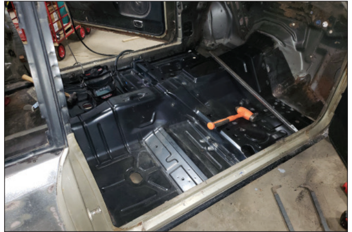
The Dynacorn floorpan has been completely welded into place and isn't going anywhere. You're going to want to scuff and primer-seal the new pan, then run body sealer around all of the seams.
