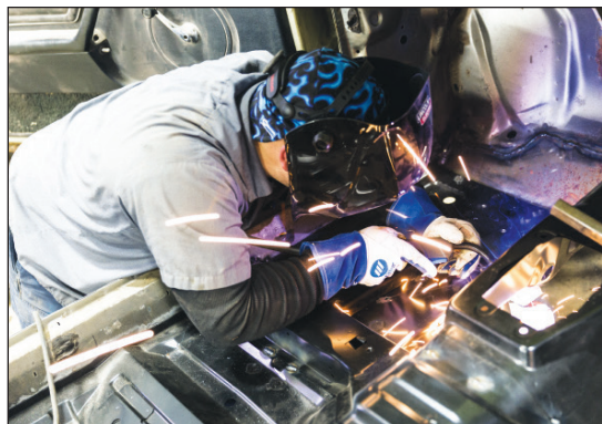
These guys are doing a terrific job of grafting in the new pan using rosette welds. Holes, approximately 1/2 inch in diameter, are drilled in the pan at the frame rail extensions and the fore and aft pans where seams overlap. These holes are rosette-welded and filled, then ground smooth until they vanish.
