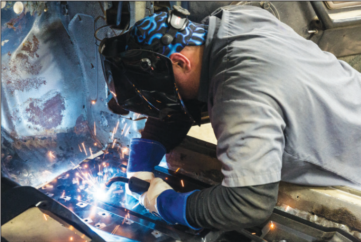
Can you see the 1/2-inch-diameter holes at the frame rail extensions for rosette-welding? This process makes the seam more solid than the factory seam.
